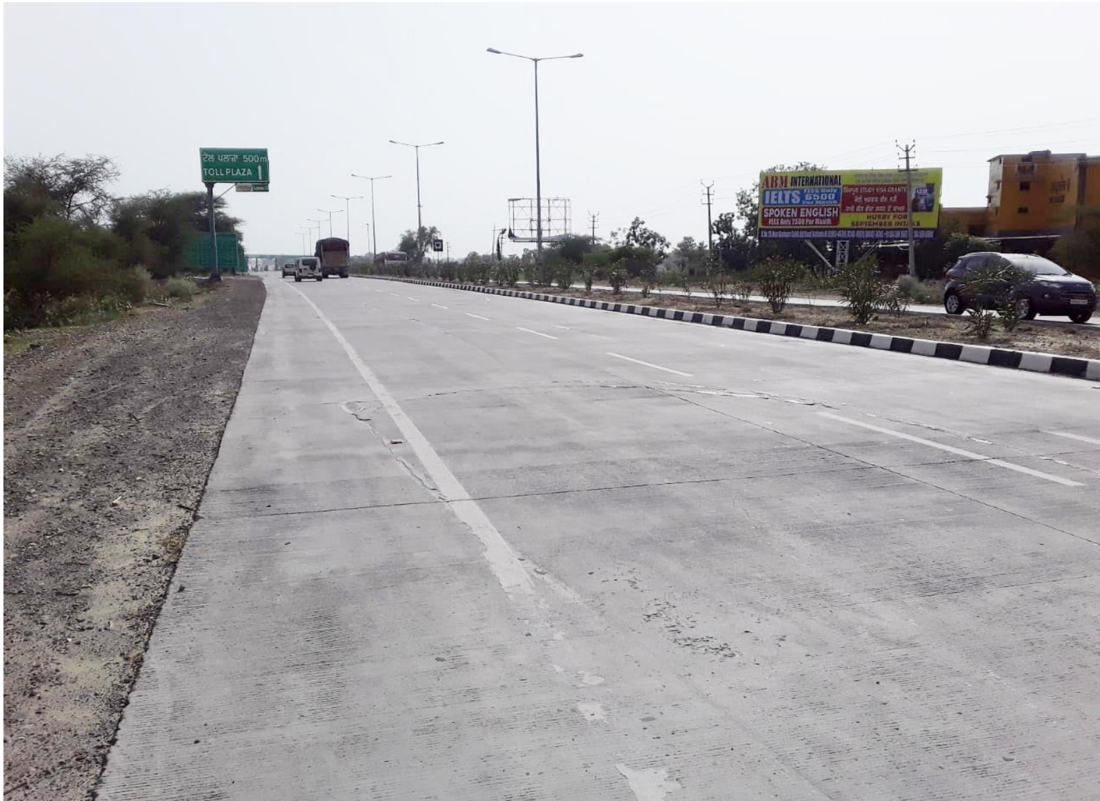
BATHINDA-CHANDIGARH ROAD NR TOLL PLAZA FCG SANGRUR, 40X16
