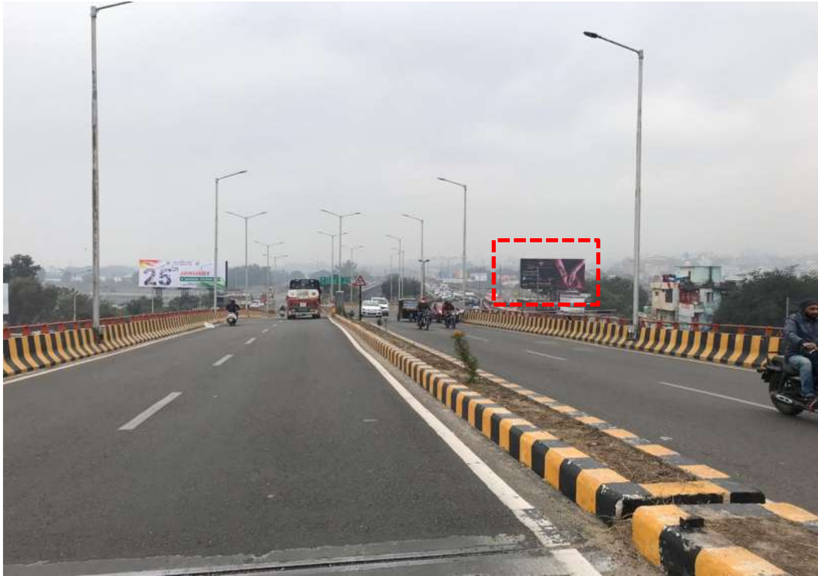
40x20,Tawi Bridge Flyover fcg Gandhi nagar Jammu
